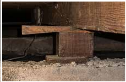
Excessive Shimming
