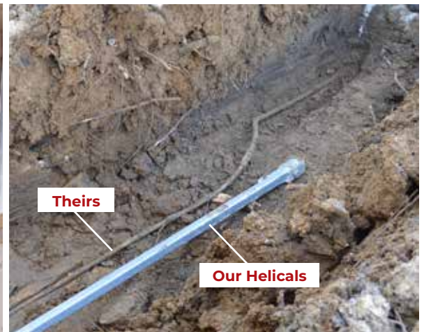
Our System - 1.5" steel extension that extends to the inactive zone
