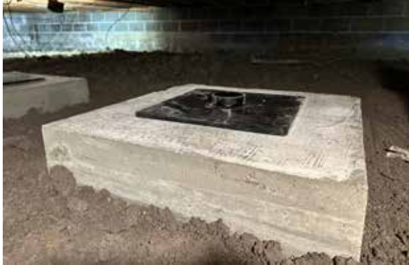
Poured Concrete Base
