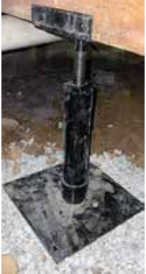
Compacted Rock Base
