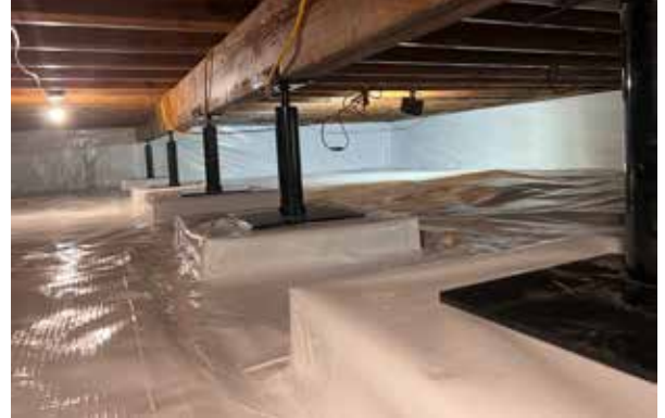
Completed Project with Encapsulation
