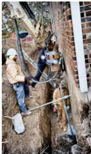
Underpinning Installation
