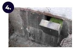
Remove section of the foundation wall.
