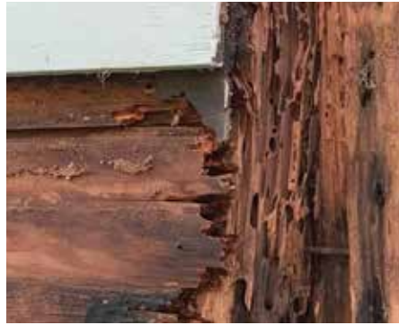
Pest infestation including wood boring insects.
