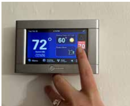
Higher utility costs due to moisture control issues.
