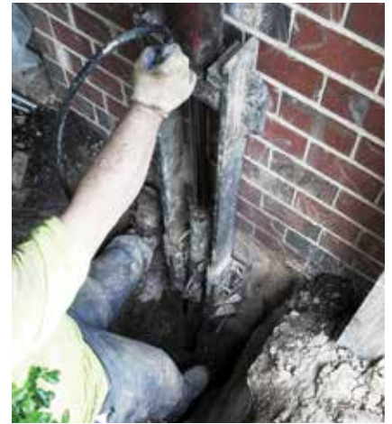
UNDERPINNING INSTALLATION
