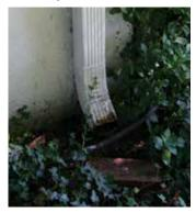
Poor drainage is a major factor contributing to expansive soils due to over saturation.
