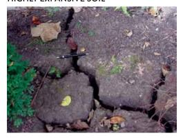
An unstable base for your home's foundation will result when expansive soils contract or shrink when moisture evaporates or drains from the ground.
