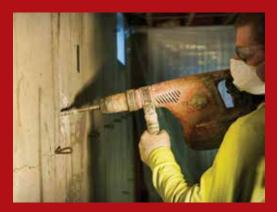
Prom the inside, extension rods are inserted through the wall where on the outside, a helix is attached. The helical anchor is hydraulically rotated into the soil at downward angle until proper depth and torque is achieved.
