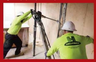
After the installation of the anchor, a threaded extension is used to connect the terminating plate or steel c-channel to secure the wall.
